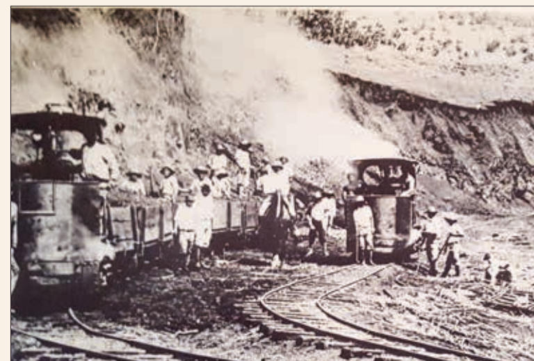
Waitā Reservoir being built in 1905.
